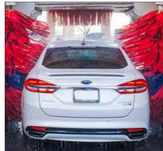
Automatic Car Wash Bay
